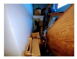
**Boiler, mechanical, and electrical panel rooms shall not be used for storage**. Combustible materials in these equipment rooms often get put too close to sources of heat and a fire may be the end result.
