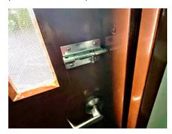
**Fire doors clear of obstructions and operate properly**. Fire and smoke doors should not be blocked open or obstructed or fire and smoke will easily travel through the opening and cause excessive risk to life and property.
