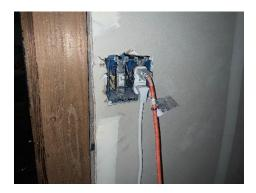
**Use of extension cords in lieu of permanent wiring is not allowed.** Temporary wire does not afford the durability, safety, and protection from shock or fire that is found in the construction of an enclosed electrical system.
